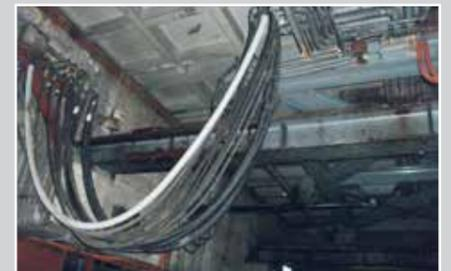
Heated hose (nominal diameter 50) for connecting storage tank and extinguishing water distribution system. Function: Protection against freezing (+ 5°C) outdoors. Material-transfer hose made of polyethylene
